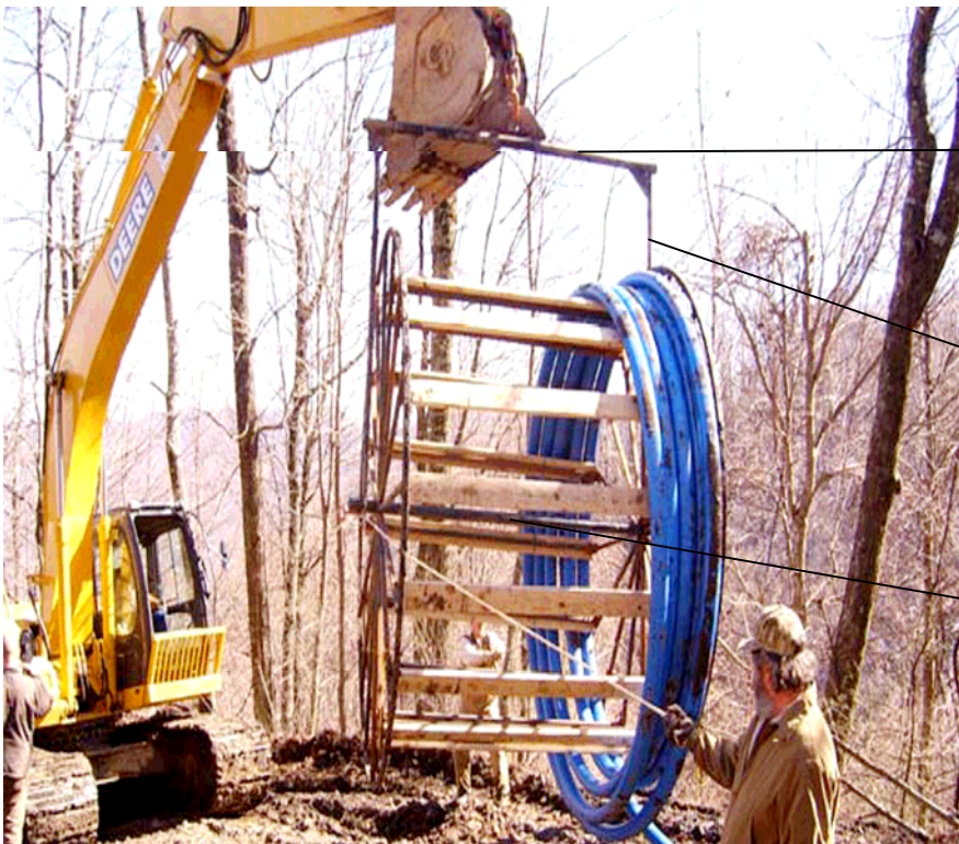
Spreader Bar. Chains or lifting Straps. Shaft
