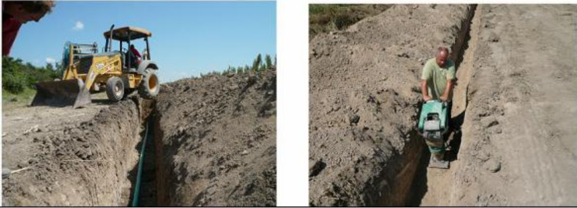
Figure 2: Backfilling and Tamping
