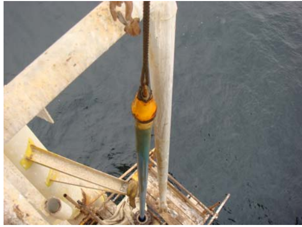
Figure 5: Tubing coming through the riser
