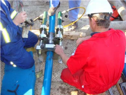
Figure 4: Splicing Tubing Together
