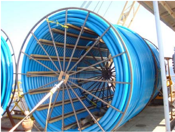
Figure 2: Spools Staged for Installation
