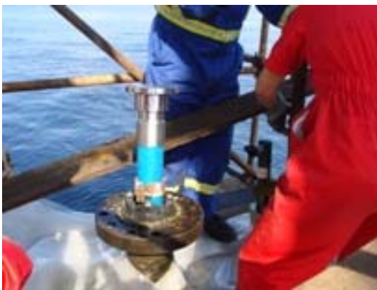
Figure 6: Flange Termination
