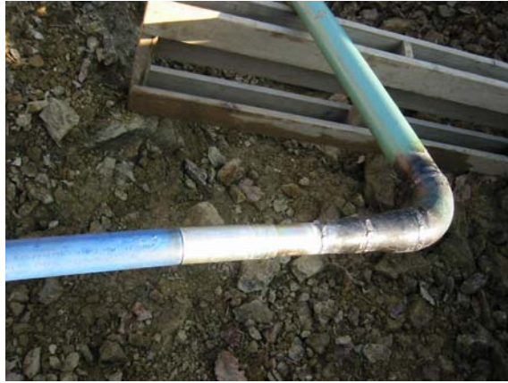
Welded Tubing to Steel Riser
