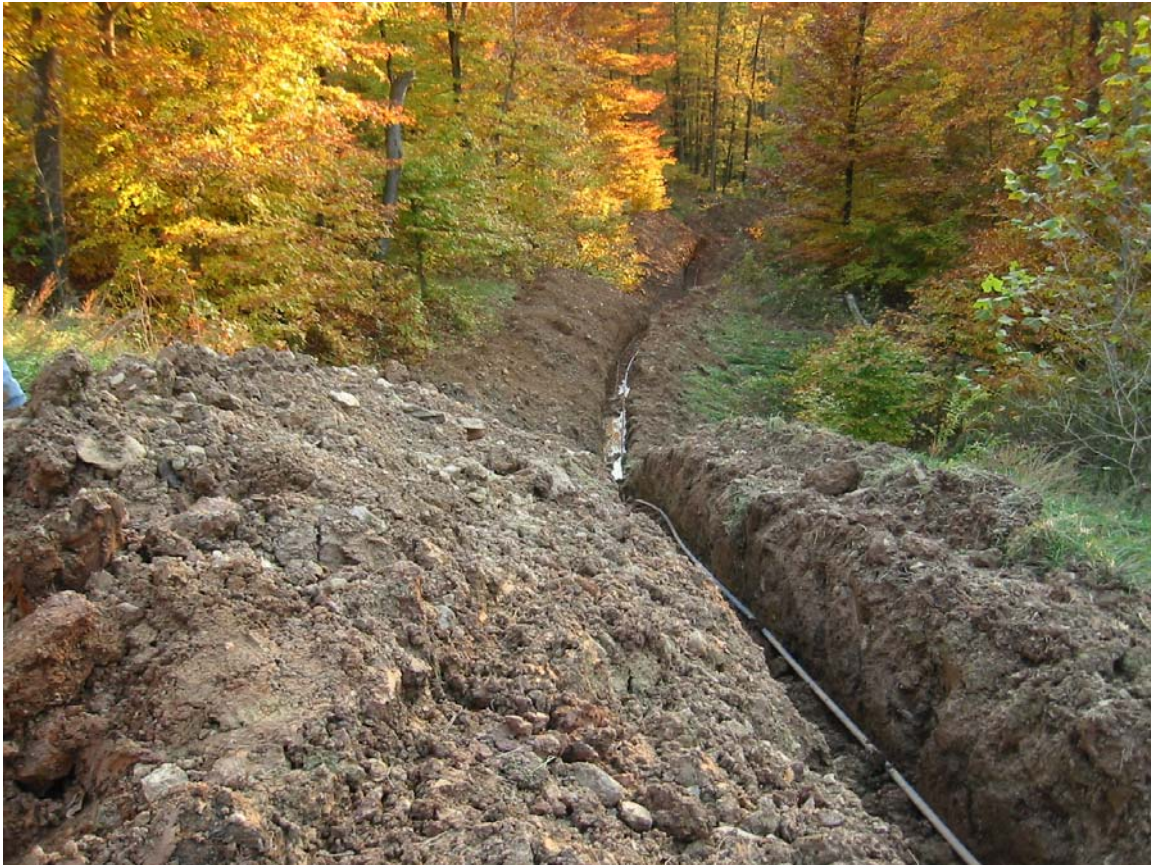
Tubing immediately after pull
