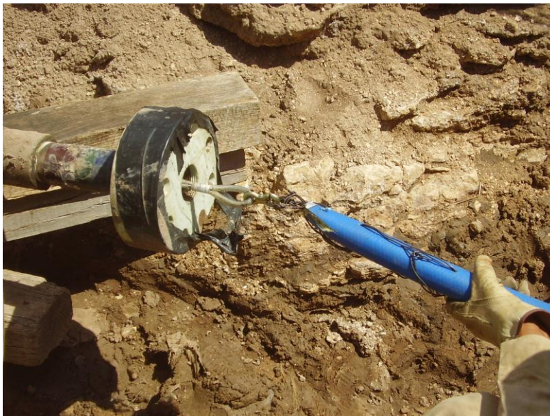
Figure 4: Feeding the tubing into the existing pipe
