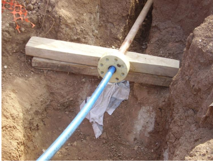
Figure 5: Pulling straight into the Existing Pipe
