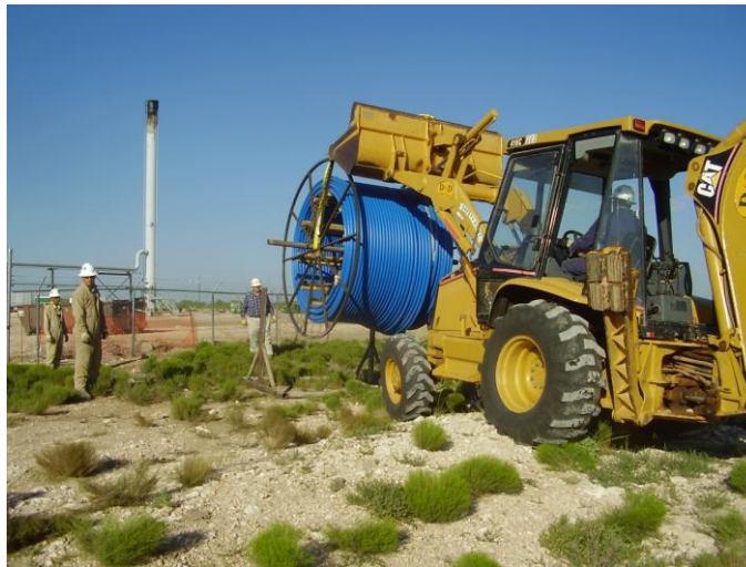
Figure 2: Backhoe setting the spool on the A-frame
