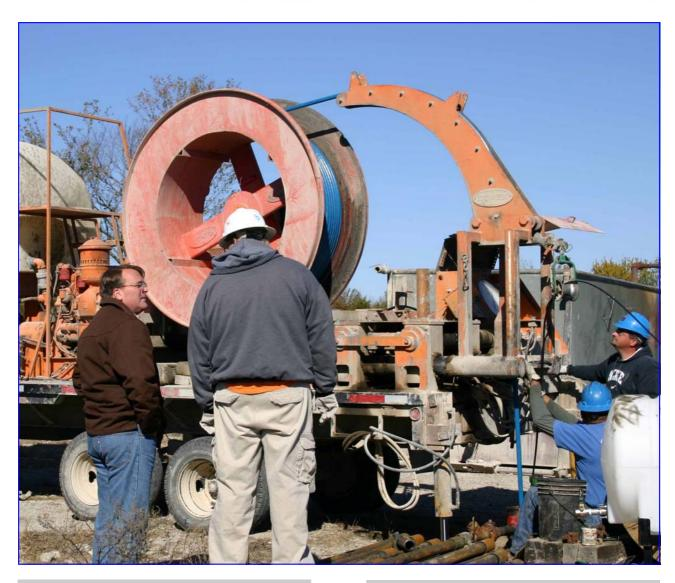
The light and highly flexible Thermoflex tube is ideal for dewatering Coal Bed Methane wells using ESP pumps: Grundfos or Smith Lift pumps for depths up to 2.000ft - 600m or Reda style pumps for depths up to 6.000ft - 1.800m.
