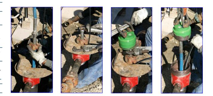
Once in position, the Thermoflex tube is held with the slotted plate and a polished rod clamp allowing disconnection from the coiling unit. The water discharge head is screwed on the tube's coupling and the power cable passed through. The discharge head is then screwed in the well head. The well head installation is further finished with the holding ring and the water discharge line with pressure gauge and sampling valve. The complete installation was executed in approx. 3 hours.
